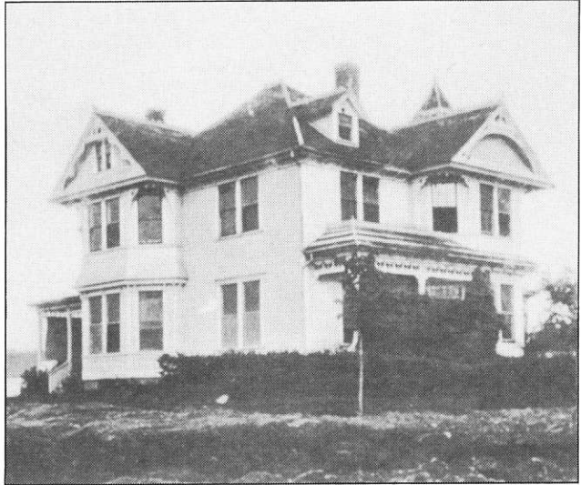
The Harris House on Bay Street; it became St. Martha's Hospital in 1907.
