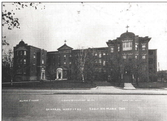
A postcard showing the old hospital with the Gibson wing completed.
