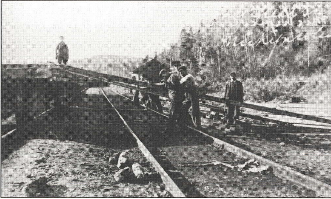
Francis Clergue mined the iron ore at Michipicoten, built a railway to carry the ore to his steel mill at Sault Ste. Marie, produced the power to run the mill, and manufactured steel rails from the ore. Courtesy SSM Museum
