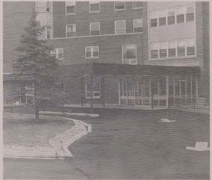
Renovations completed on front entrance.
