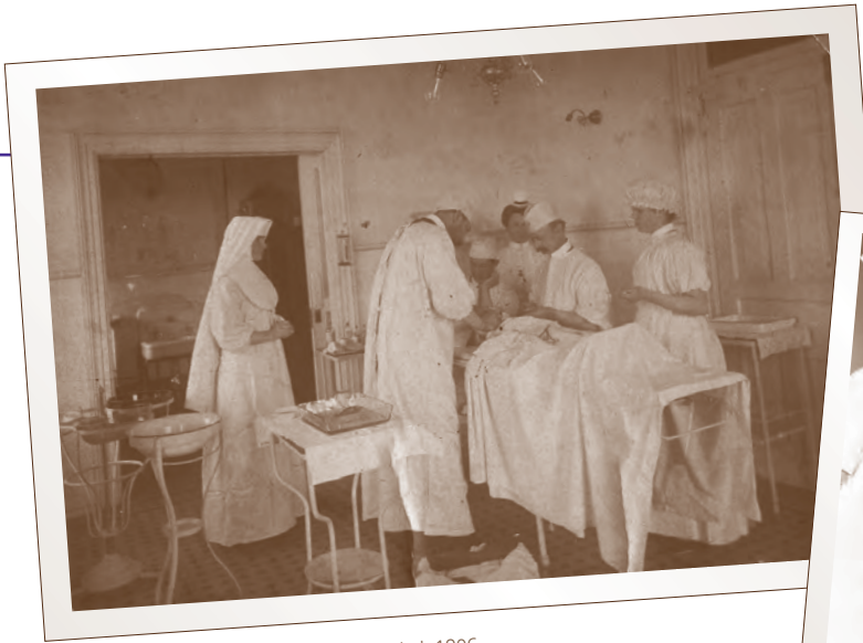
Operating Room, St. Joseph's General Hospital, 1906
