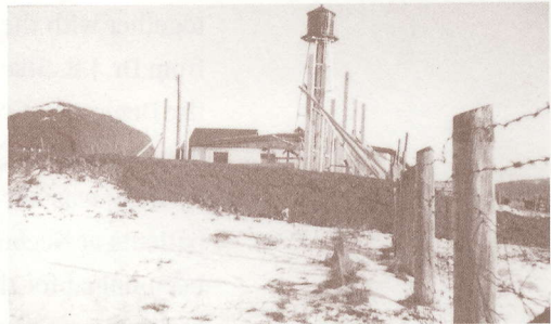
Water tower at Ontario Hospital Fort William, 1937
