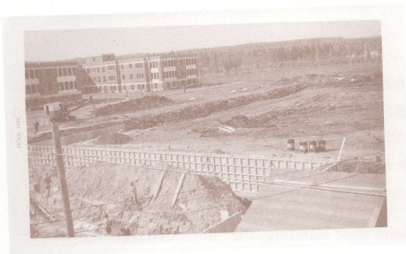
Connection between administration buildings to pavilions under construction, early 1960's
