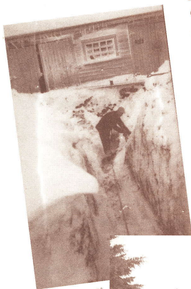
Water problems at Ontario Hospital Fort William, 1937
