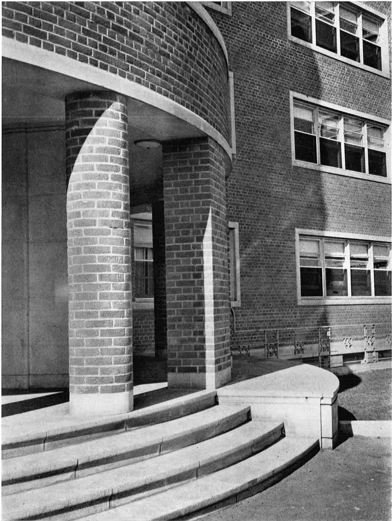
ENTRANCE PORCH DETAIL
