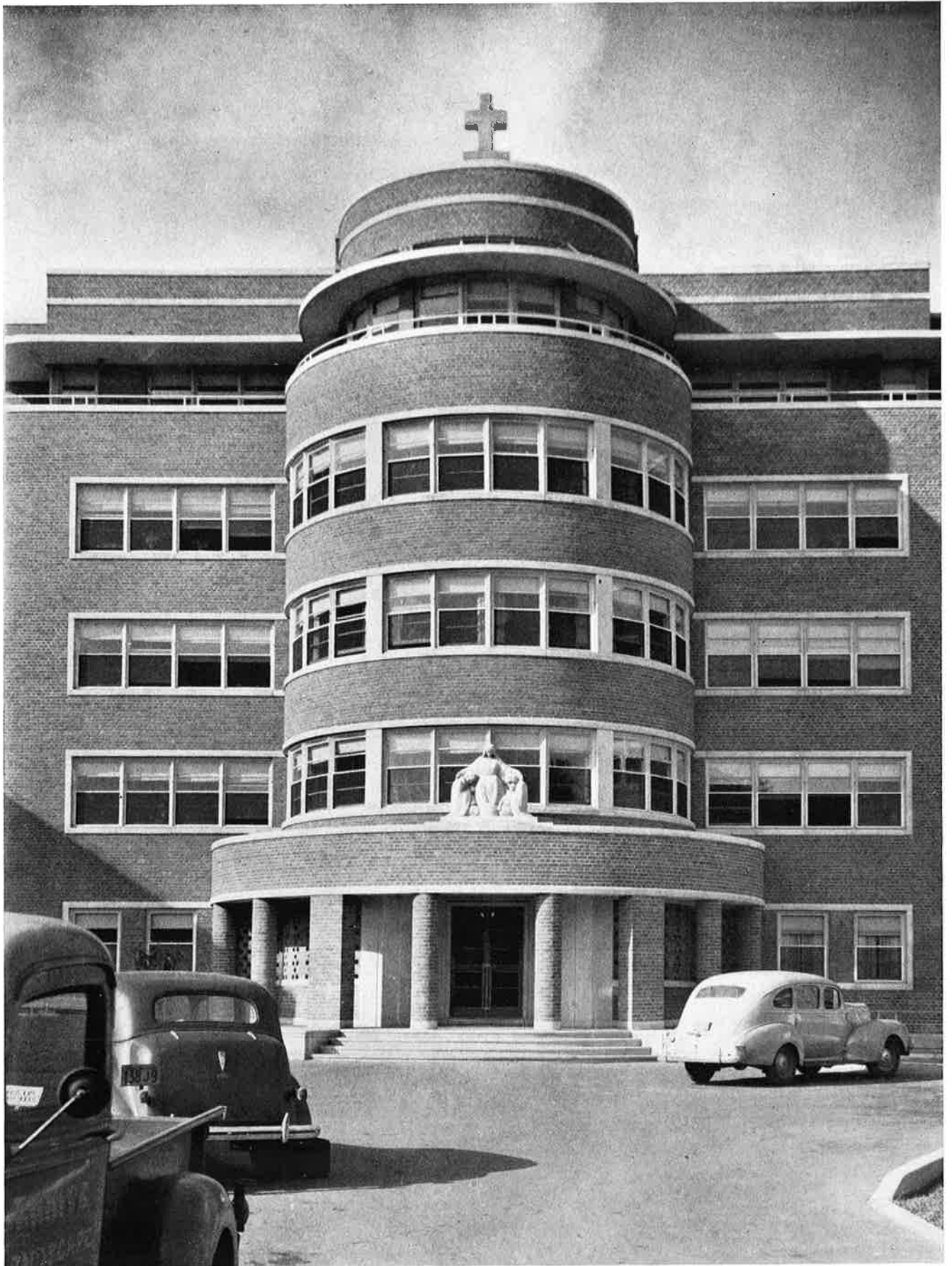
OUR LADY OF MERCY HOSPITAL, TORONTO, ONTARIO MARANI, LAWSON AND MORRIS, ARCHITECTS
