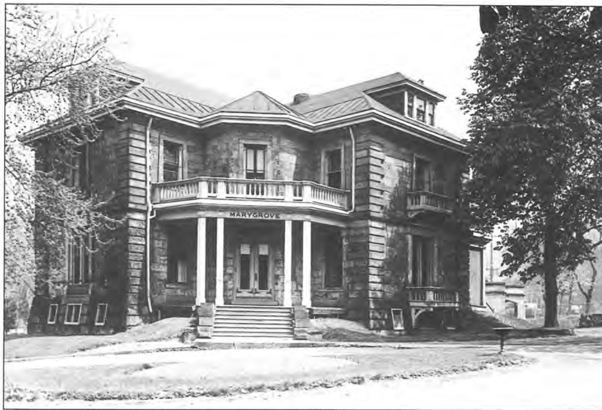
Marygrove was built in 1869 at the corner of James Street South and St. Joseph's Drive. The hospital purchased Marygrove on September 15, 1947, for use as a nurses' residence. In 1960 it was demolished when construction of the new surgical building began.
