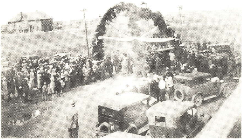
Opening of the road. Railway station at Hearst in the background
