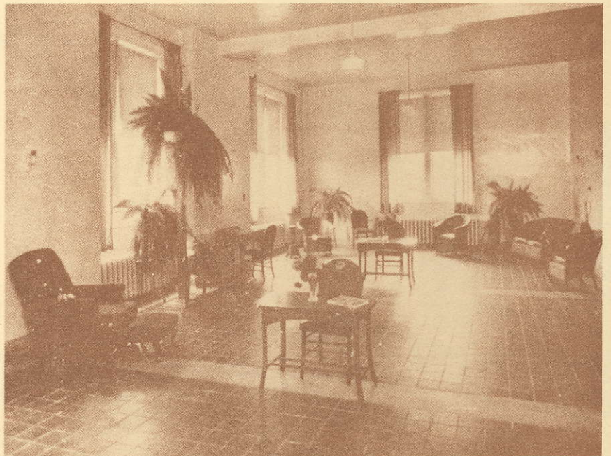
1935: Solarium in St. Joseph's Wing. There was one on each floor.
