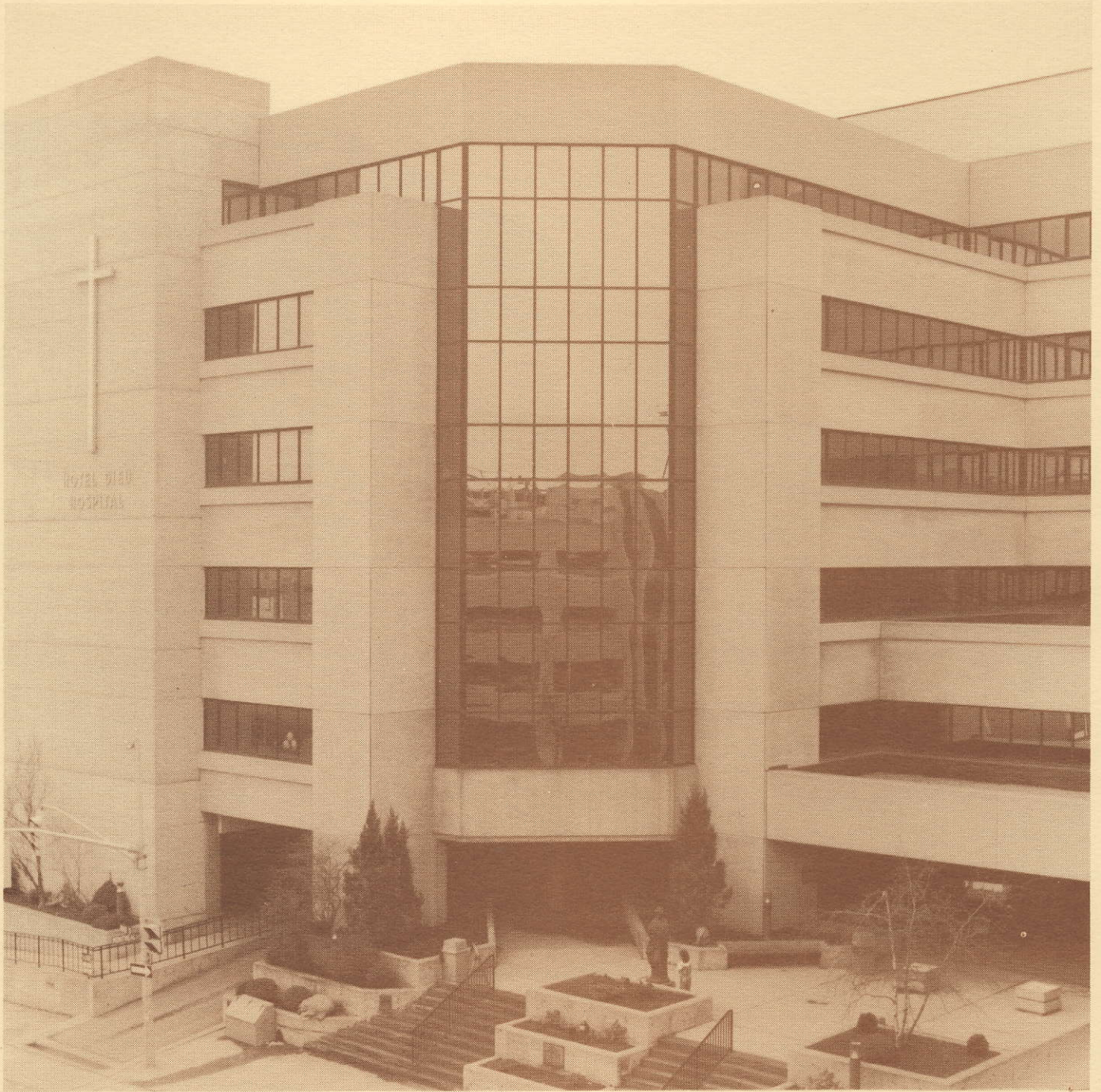
Hospital's main entrance on Brock Street.
