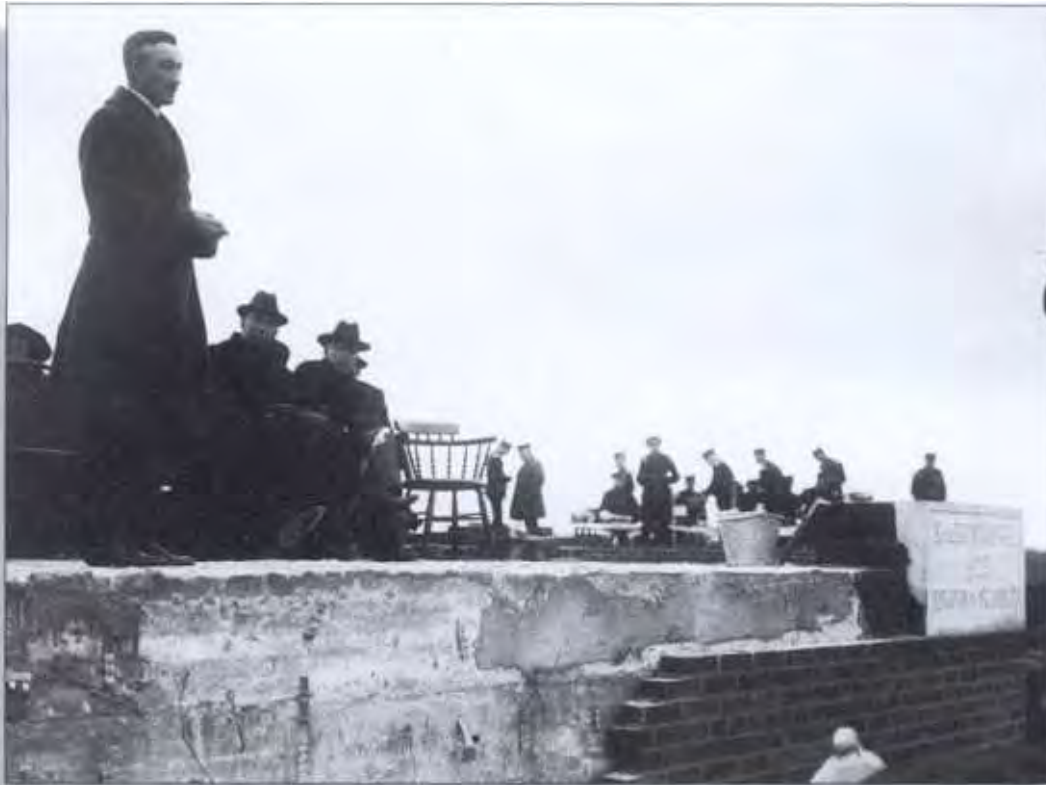
Kitchener mayor (and future Ontario Lieutenant-Governor) Louis Orville Breithaupt speaks at the hospital's corner- stone laying. Despite later additions to St. Mary's, the original cornerstone is still visible just outside the hospital's emergency entrance. Source: SMGH
