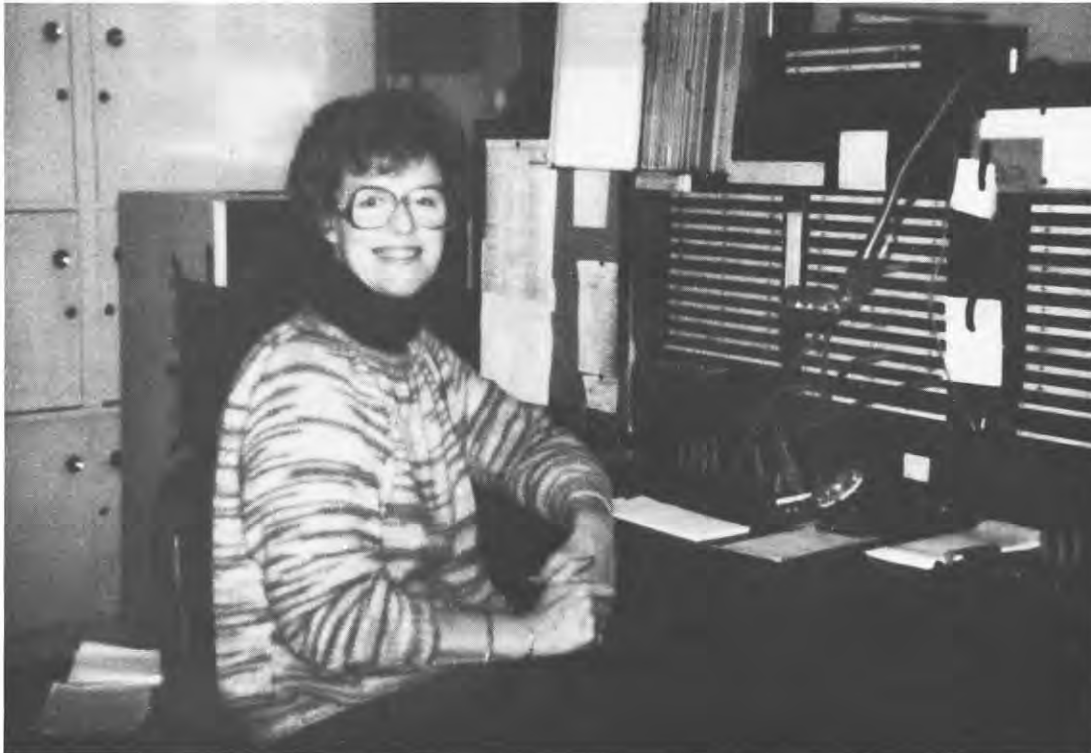
A mid 1970's view of the Cord-type Switch-board with operator Sally Rice.
