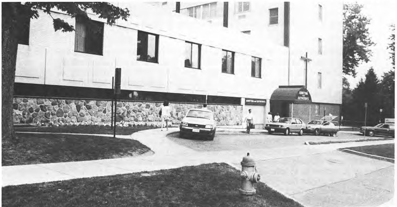
The entrance to Admitting and Out-Patient facilities is reached from this semi-circular driveway off Grosvenor Street. The large windows on the first floor are in the Coronary Care Unit.
