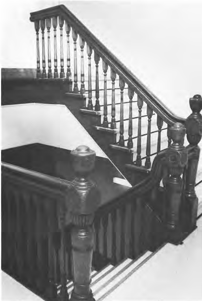
The only remaining portion of the 'Grand Stairs' as viewed from the third floor. Fire regulations required the lower portion be removed in the 1950's.
