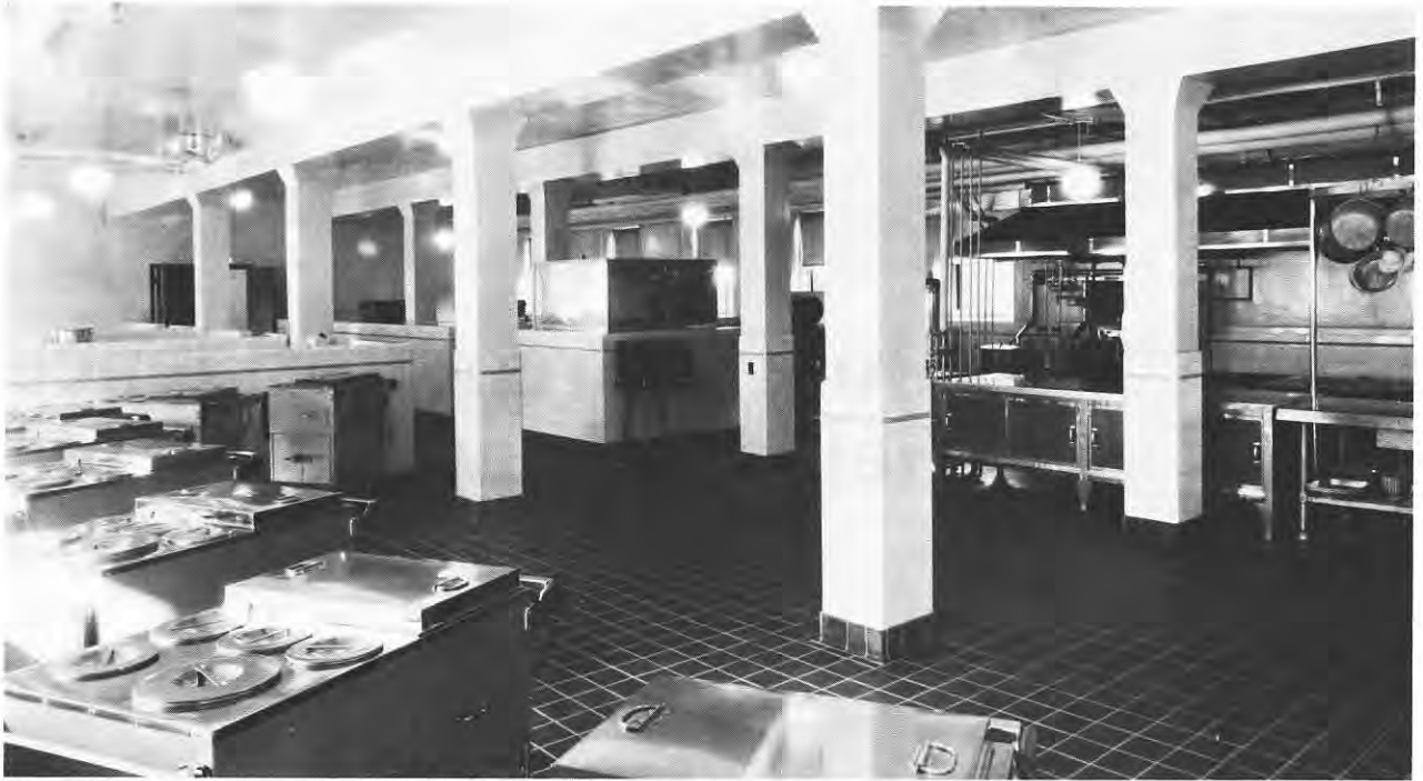
The new Kitchen with areas for specialized preparation to the left.
