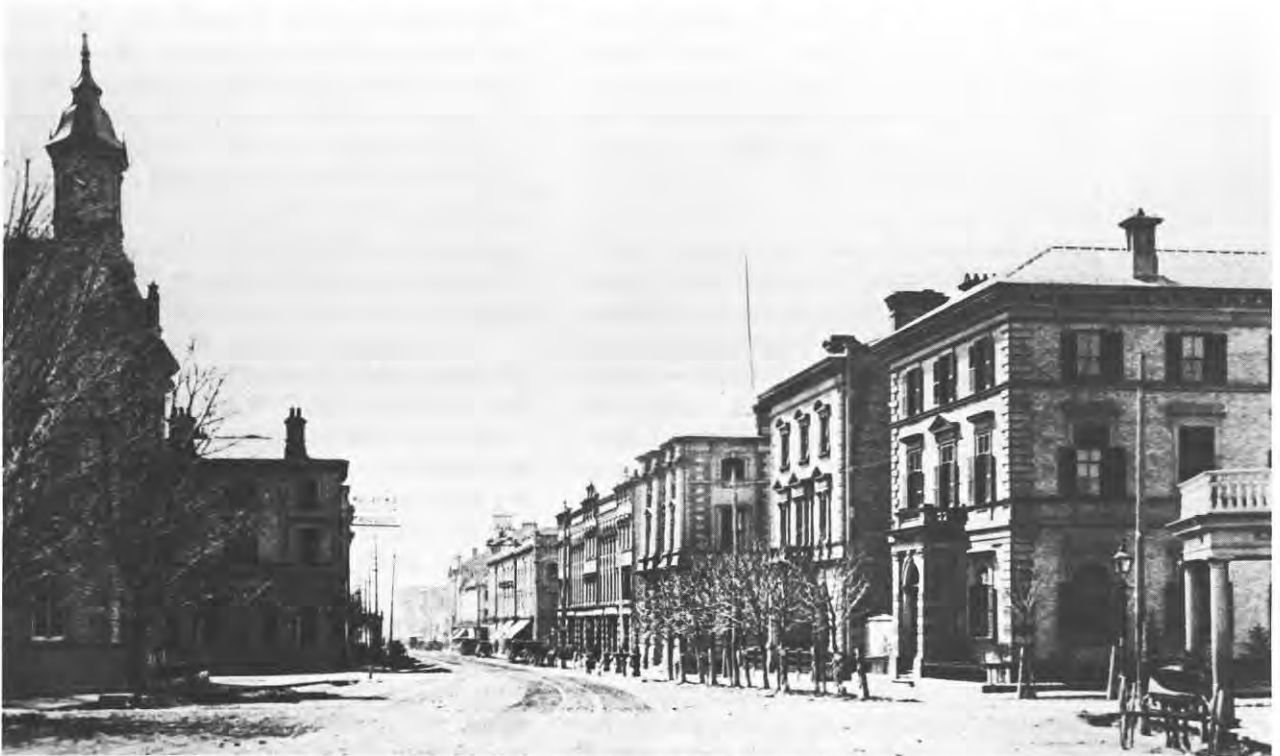
Richmond Street looking south from St. Paul's Cathedral circa 1875. The right foreground shows the Bank of Montreal and Merchants Bank, between Fullarton and Queens Avenue, on the site now occupied by the Federal Building. Just beyond is the Post Office, now the Bank of Montreal. On the left is the Customs House, now lawn area of St. Paul's Cathedral. Beyond Queens Avenue is another Bank of Montreal, now the Anglo-Gibraltar Building.
