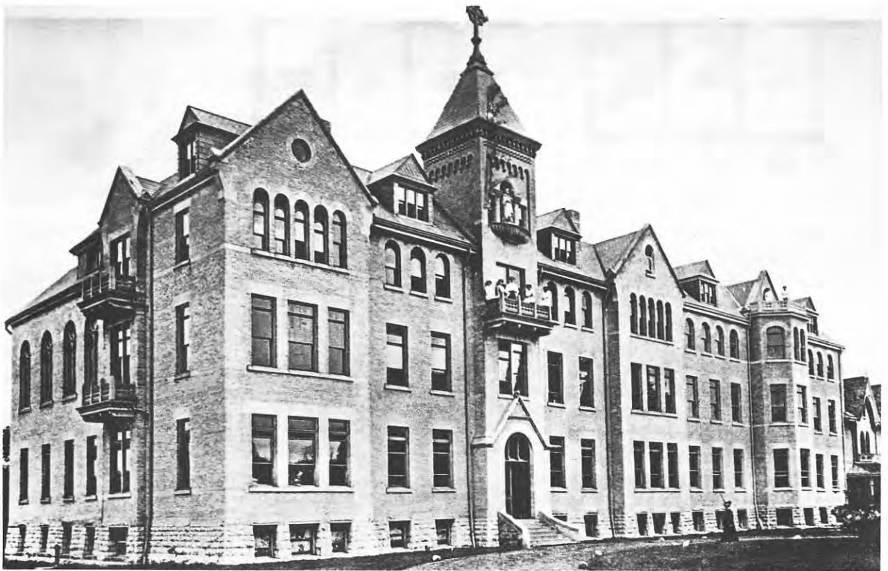
St. Joseph's Hospital 1903, including 1892 building.
