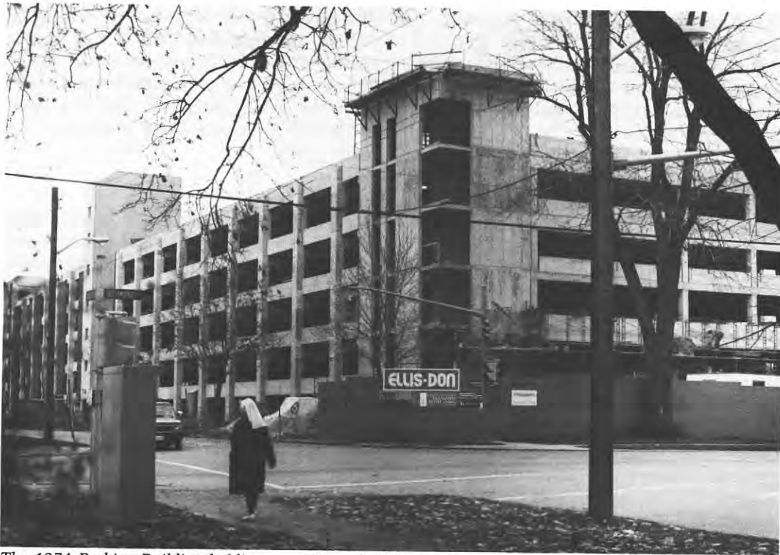
The 1974 Parking Building holding approximately 800 cars has now been augmented with space for 400 additional cars. At the Richmond and Grosvenor Streets corner of the building, facilities have been included for a connection to the tunnel which will join St. Joseph's and St. Mary's Hospitals.
