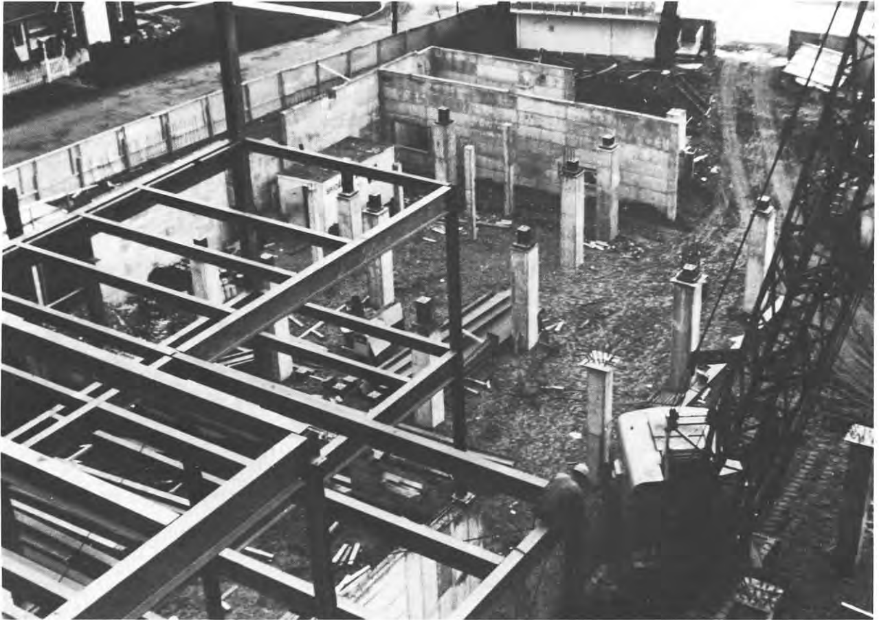
Early stages of the 1964 construction, Wellington and Cromwell Streets.
