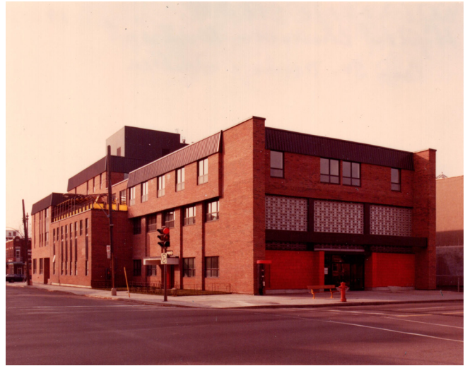
Montreal Chinese Hospital, 1965 (corner of St-Denis and Faillon Streets)
