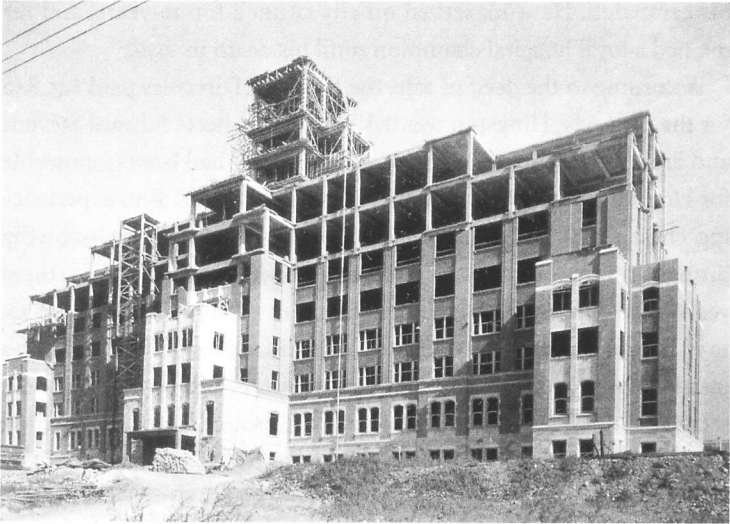
St. Mary's under construction, spring 1934. Courtesy of Dr. Richard Moralejo.
