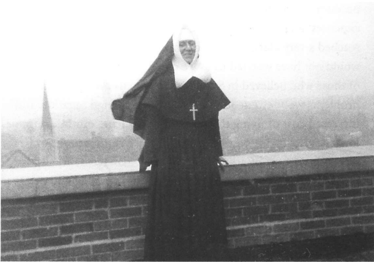
Mother Superior Mary Adalbert Rozmahel, seen here on the roof of the hospital, brought the Sisters of Providence to St. Mary's in 1943.
