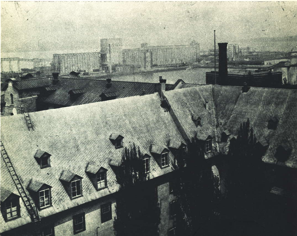
▼ Interior Court of Cloister, Hotel Dieu, Quebec, with harbour in background.
