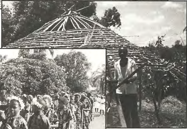
Building a tent
