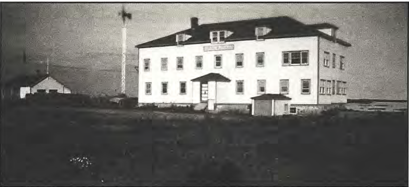
Fort Rae, Farquhar Hospital, 1940
