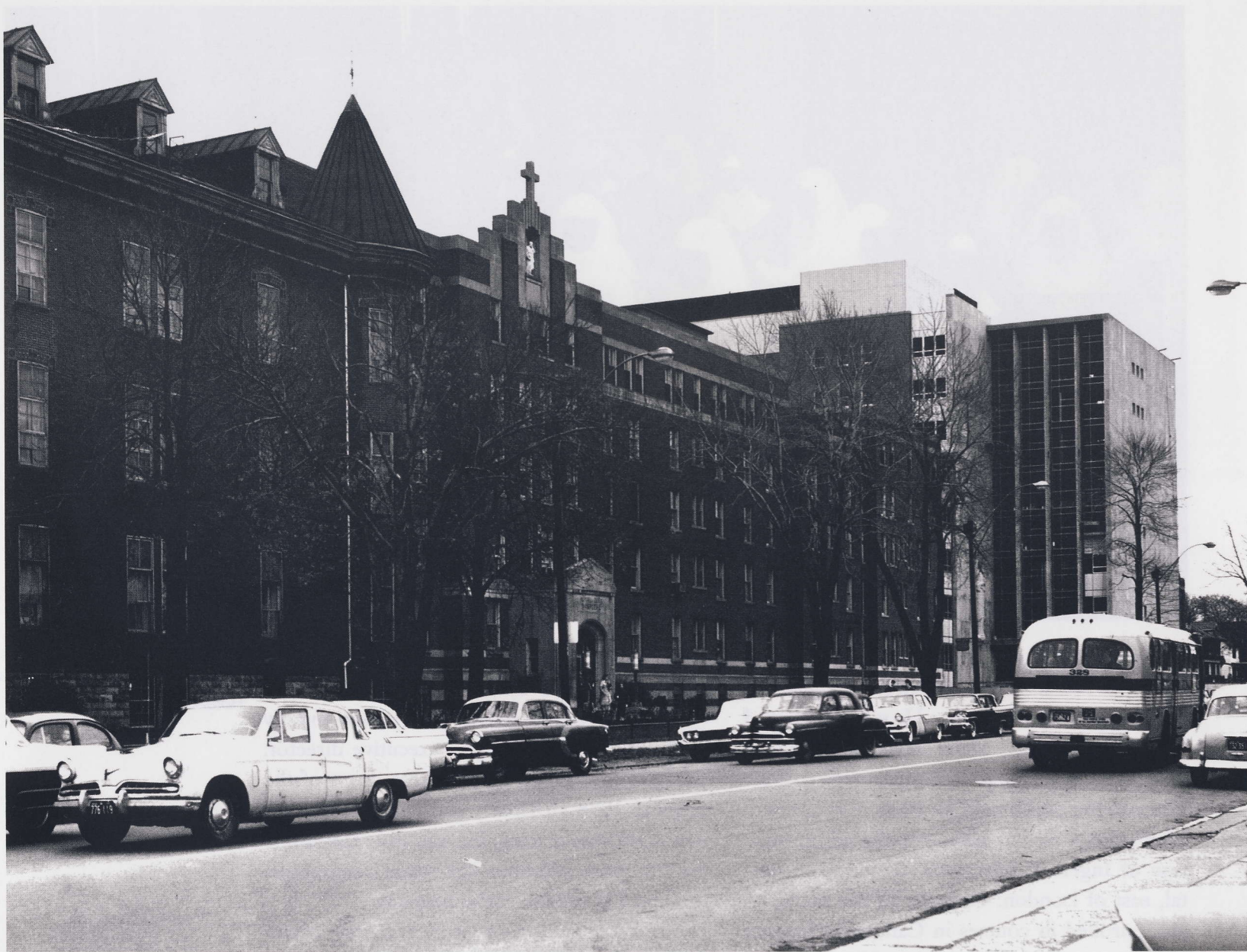
Construction of 1962 wing
