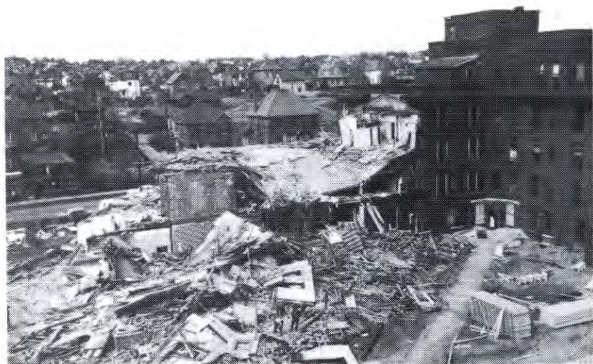
Demolition of 1884, 1900 and 1905 wings, March 1958.
