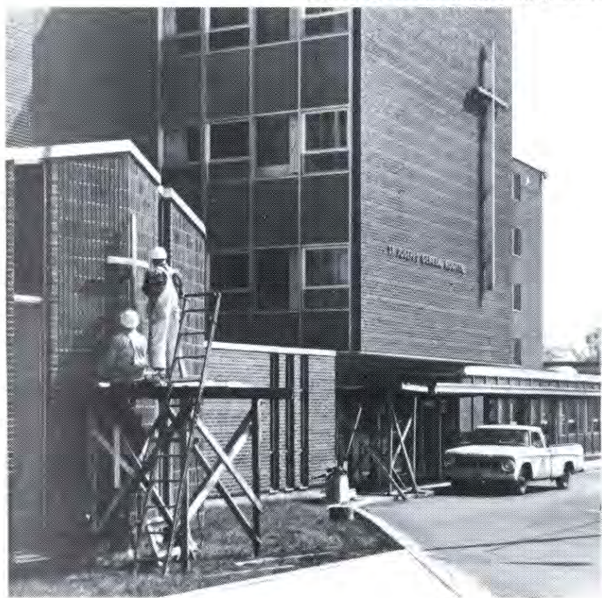
Finishing touches to new wing, 1967.
