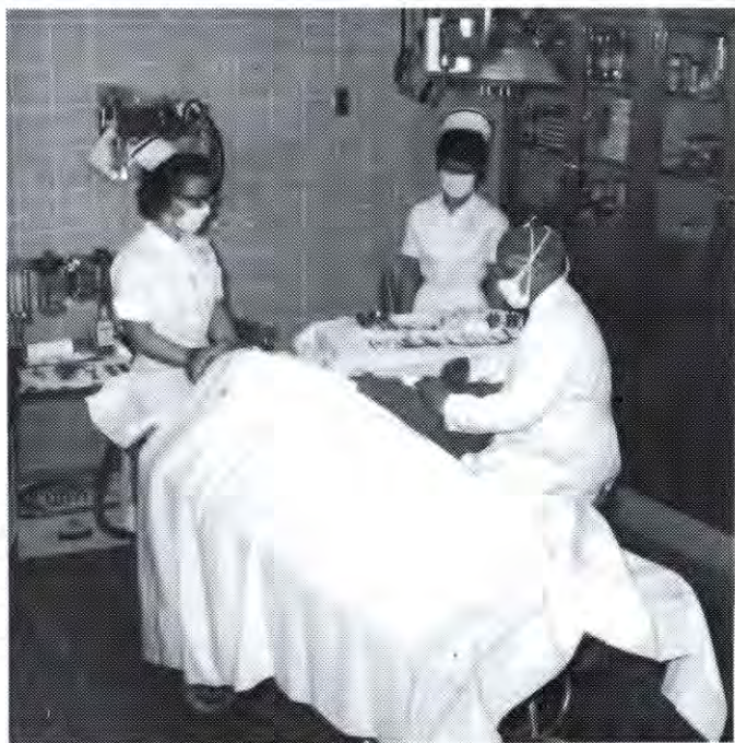
Emergency Room, 1959 wing, 1st floor, circa 1963.
