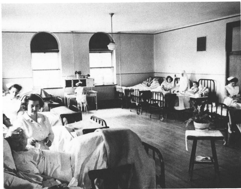
Old D-Wing ward rooms.
