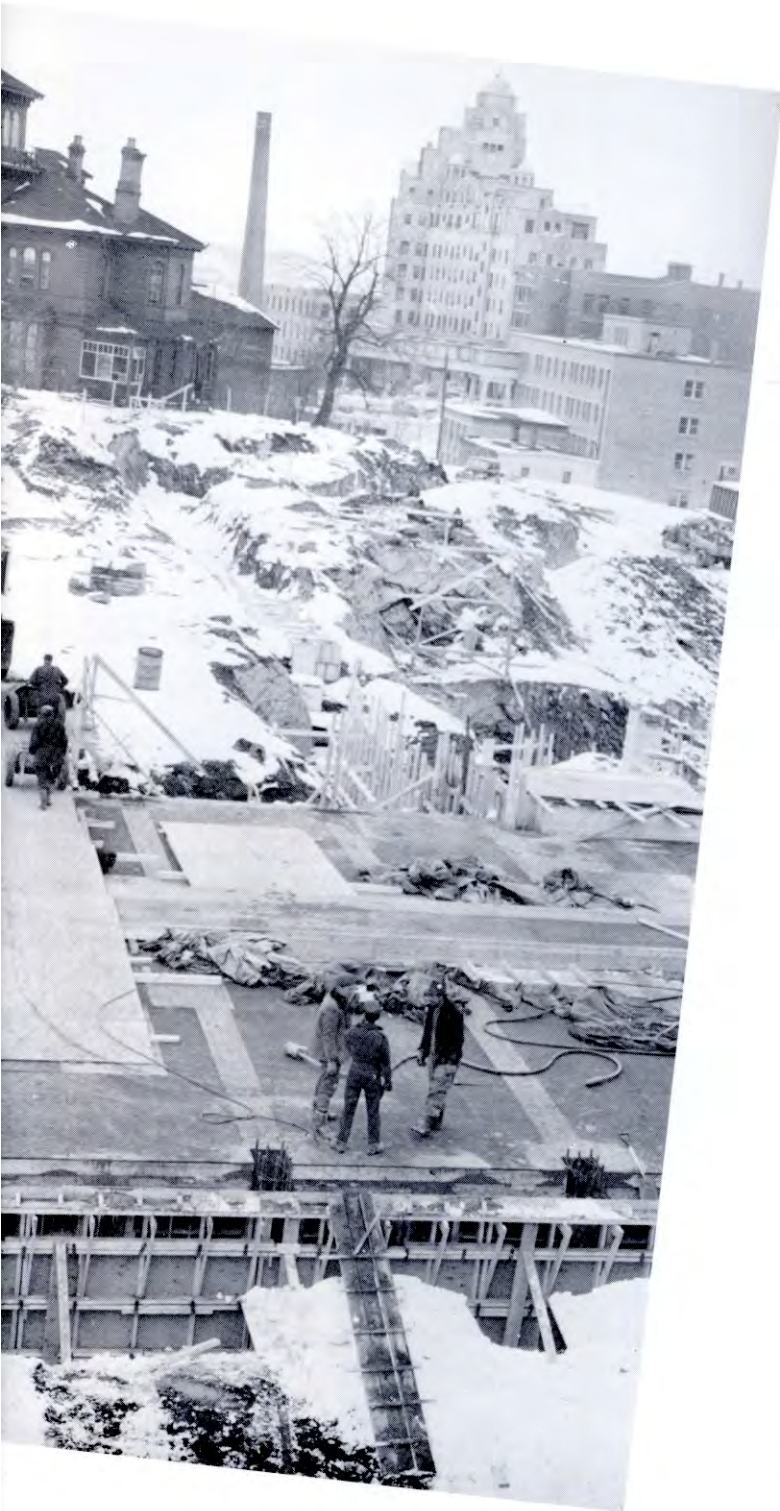
New hospital under construction. Hazen home shown in background.
